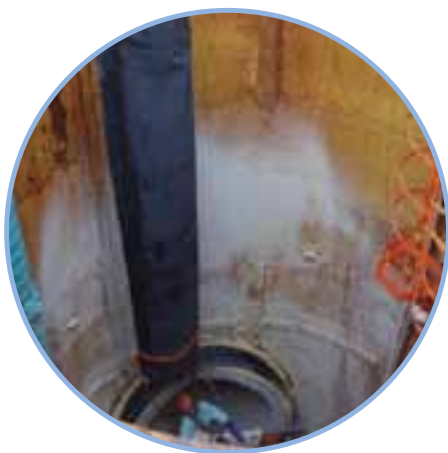
Inserting a folded pillow plug
