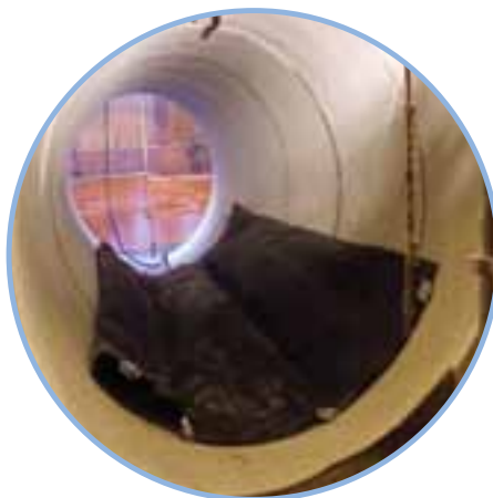
Placing – pillow plug should be positioned horizontally
