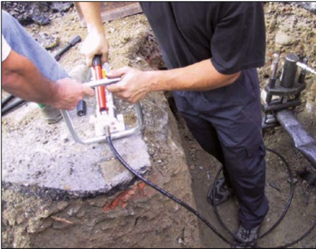
Pumping operation for pipe compressing
