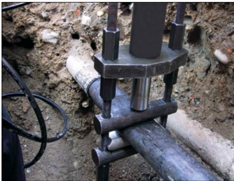
Pumping operation for pipe compressing
