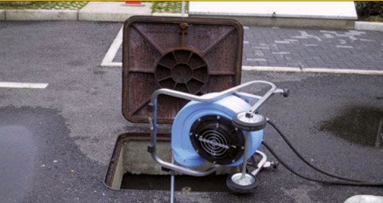
Ventilation positive and negative
